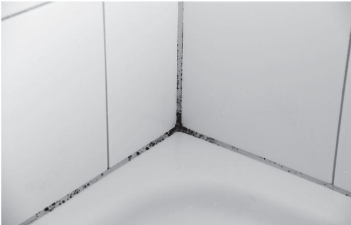
Mold on silicone joint in the bathroom
